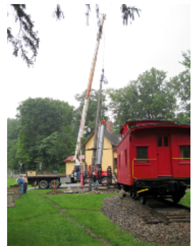
Installing the Signal
