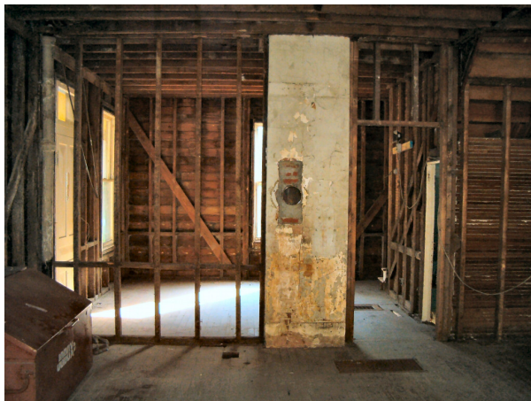
Daylighting the studs
