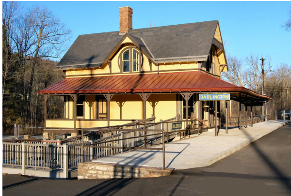
The station in November 2007 after exterior restoration
