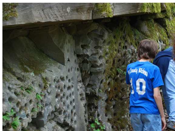
Test drill holes, A.k.a. Swiss cheese wall
