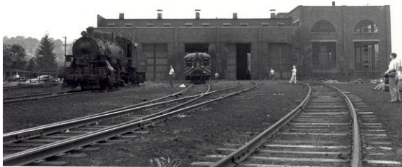
This photograph taken before 1952 shows the LVRR engine house on the north side of Main Street while still in use.
